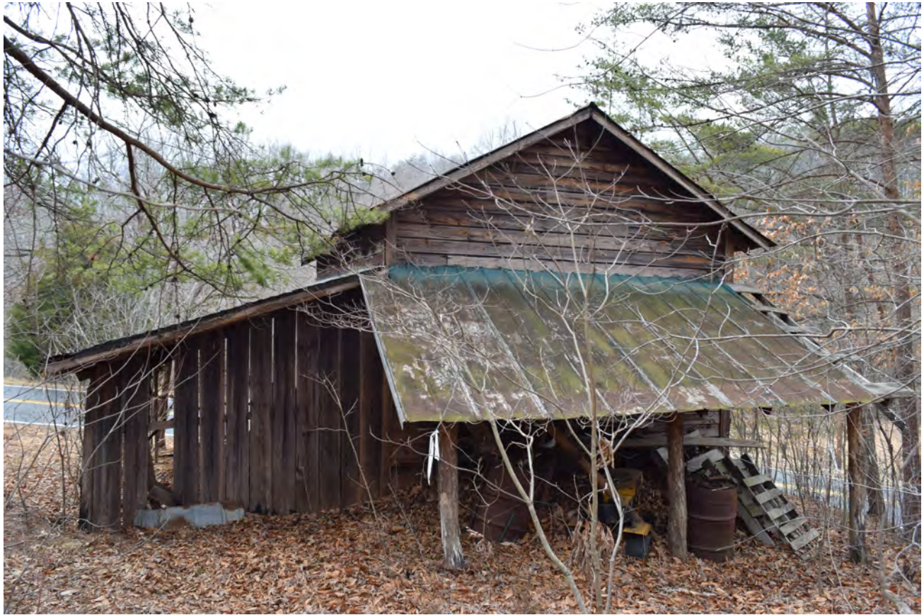
Figure 22: East side of pack house, facing west
