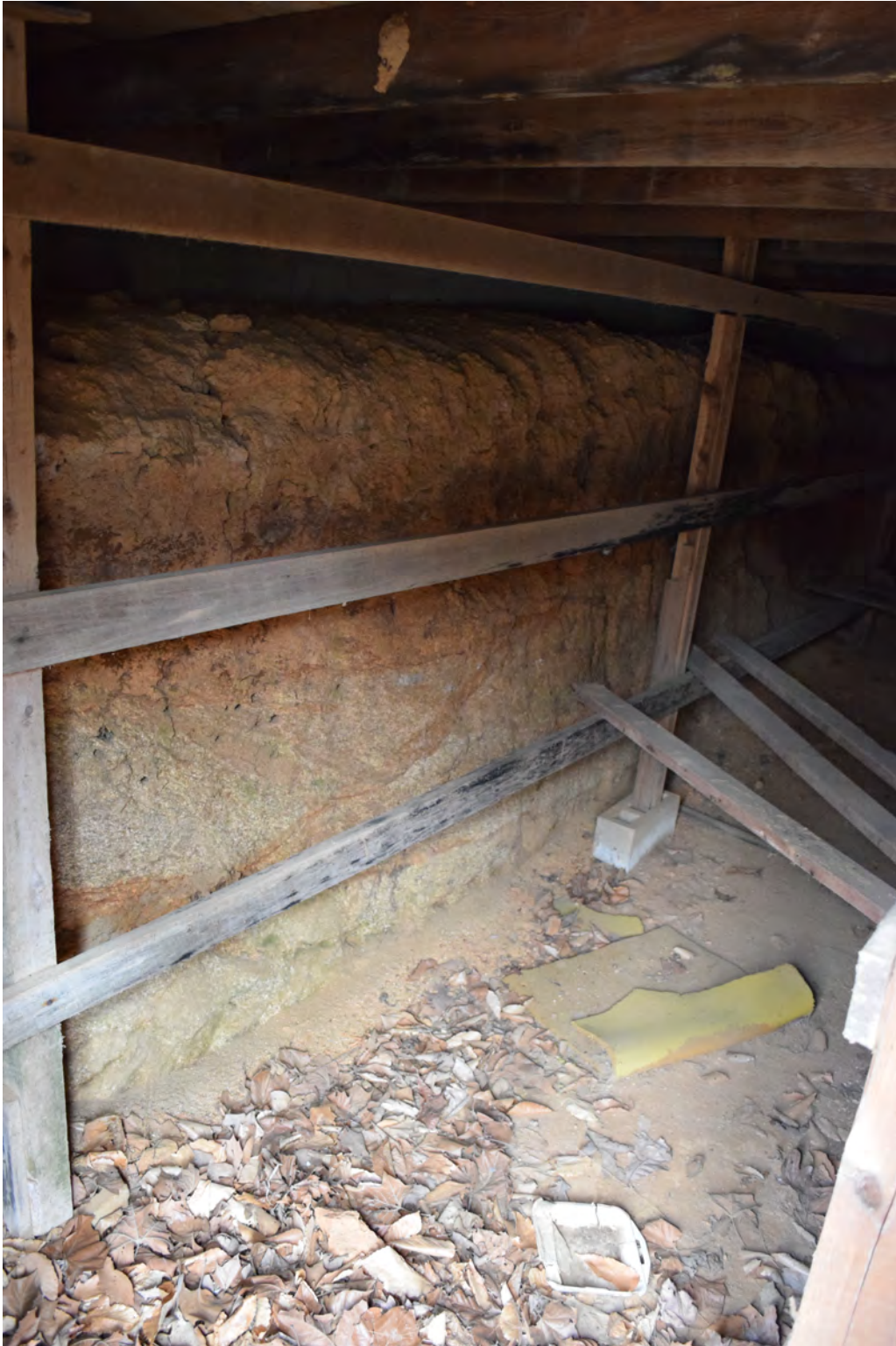
Figure 23: Granite walls in pit basement of pack house, facing northeast
