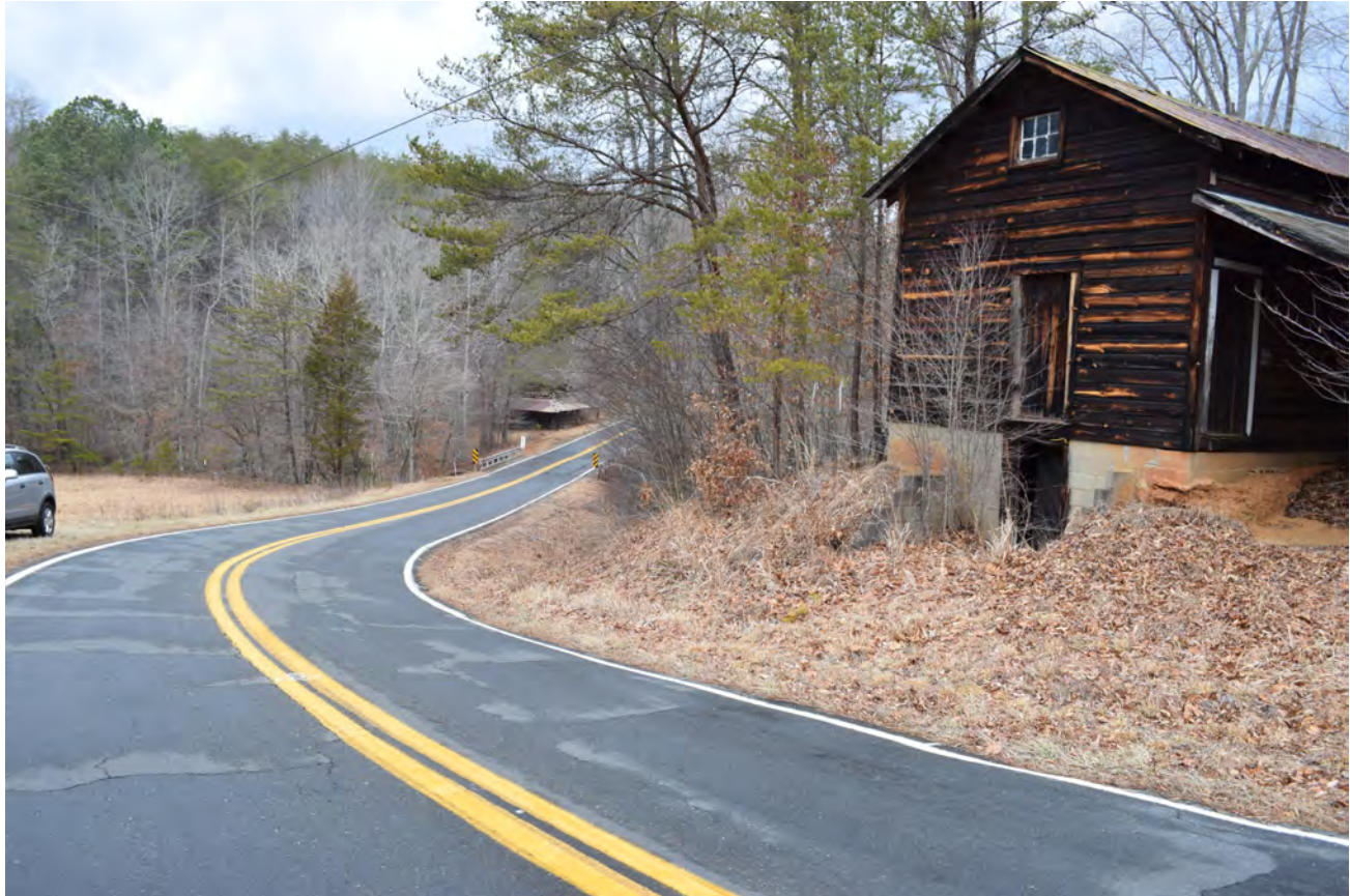
Figure 8: Pack house southeast of bridge and on the east side of Tom Shelton Road, facing north-northwest
