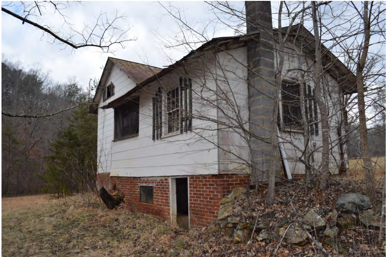
Figure 10: Tom Shelton House, southwest corner of kitchen addition, facing north-northeast
