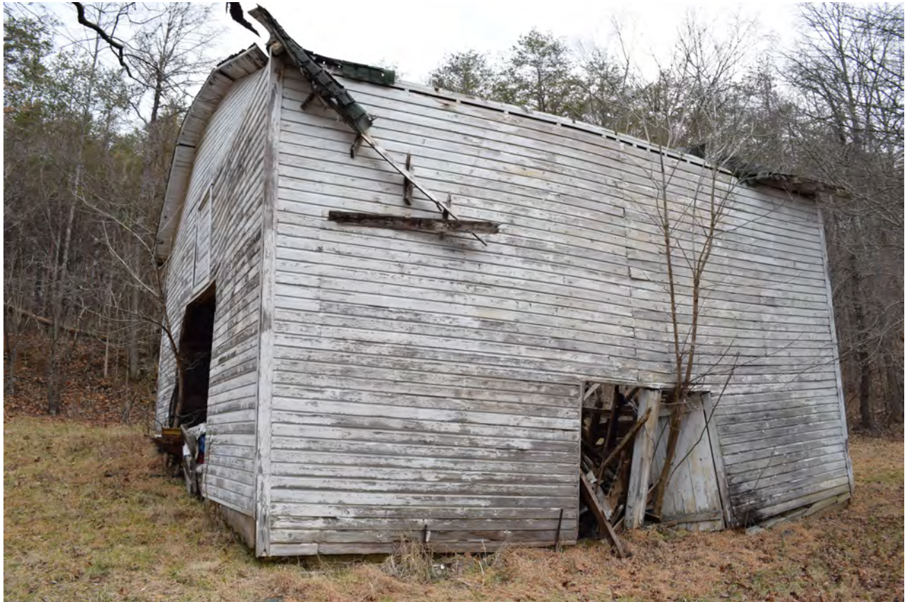
Figure 19: Barn, west elevation, facing east
