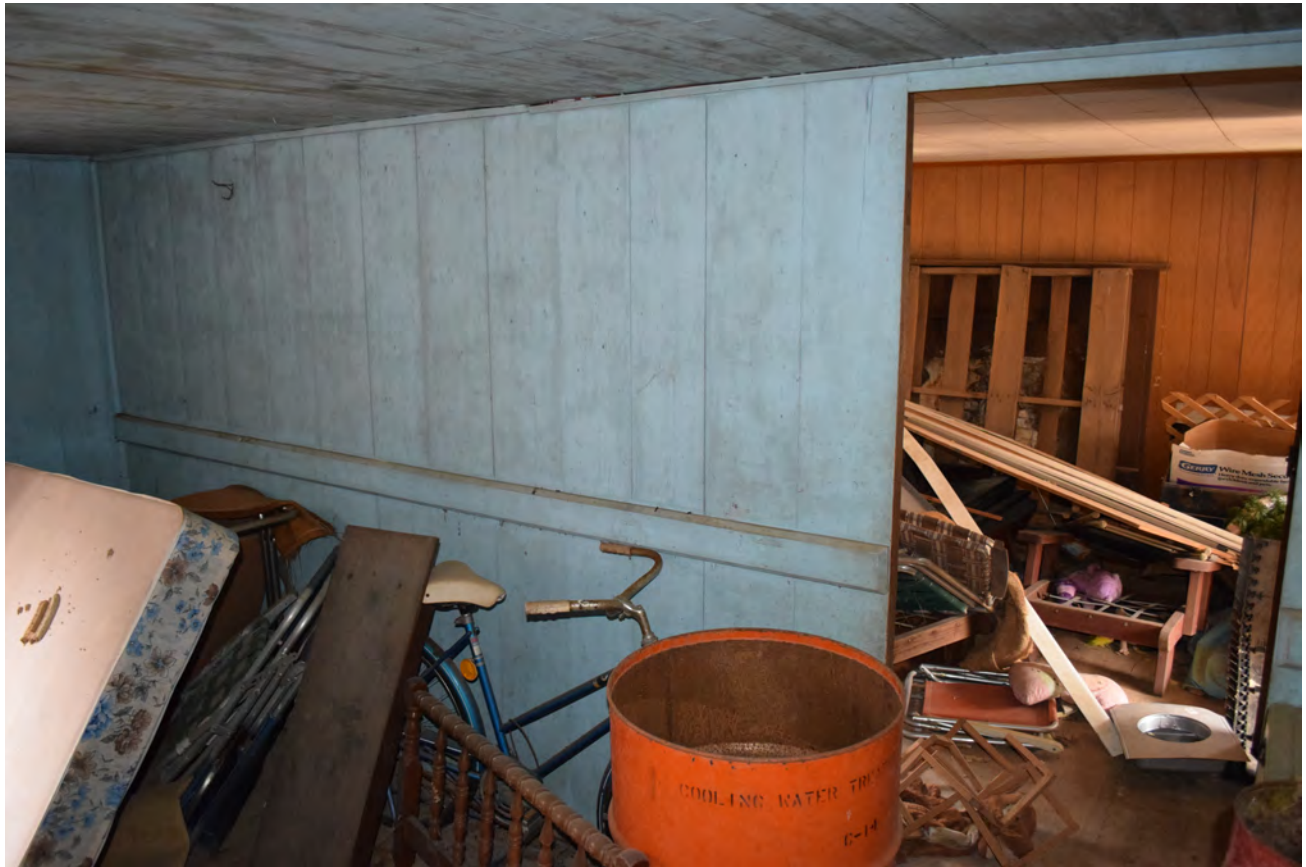
Figure 13: West room in Tom Shelton House, facing north-northeast
