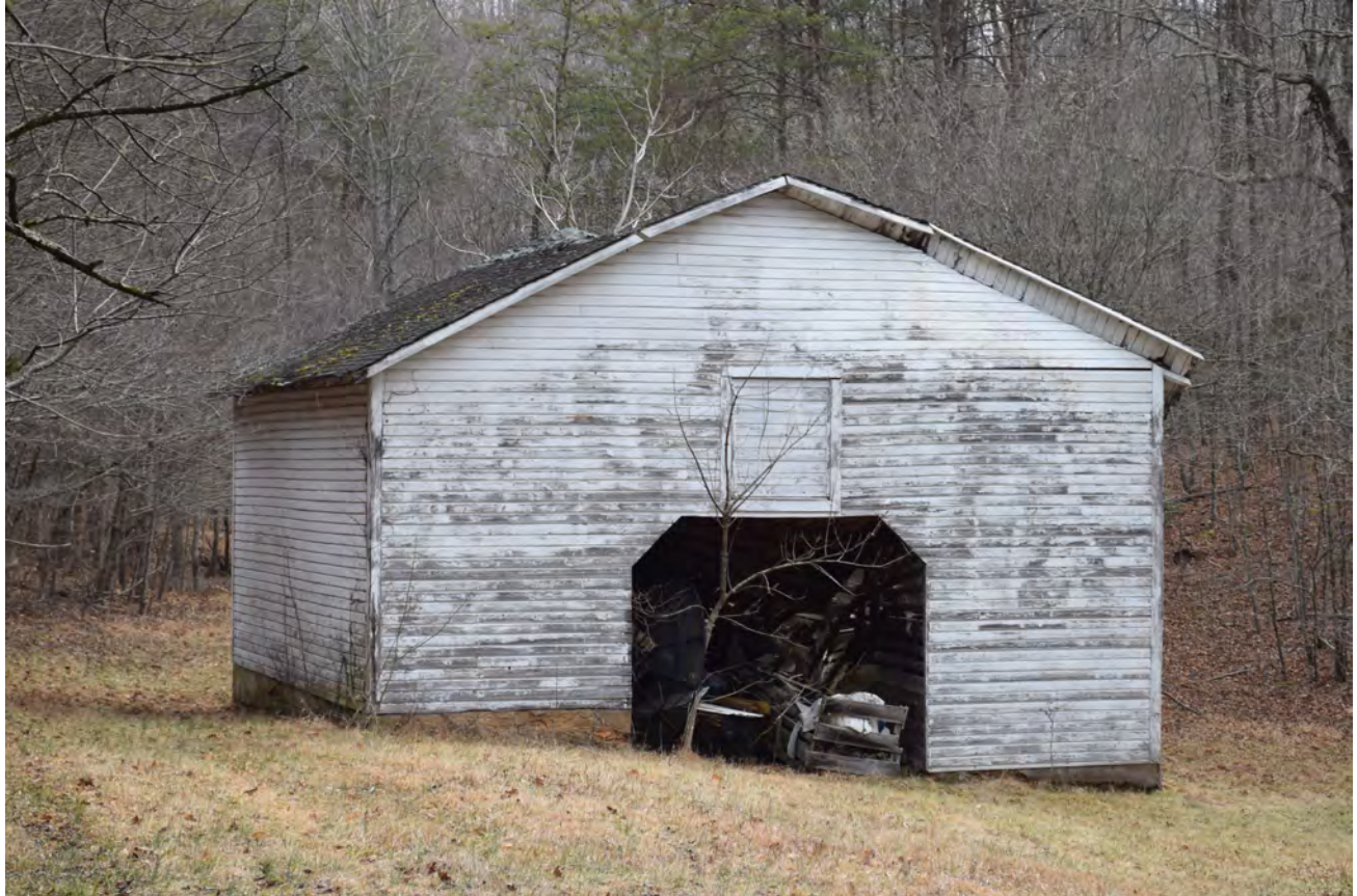
Figure 18: Barn facade, facing south-southwest
