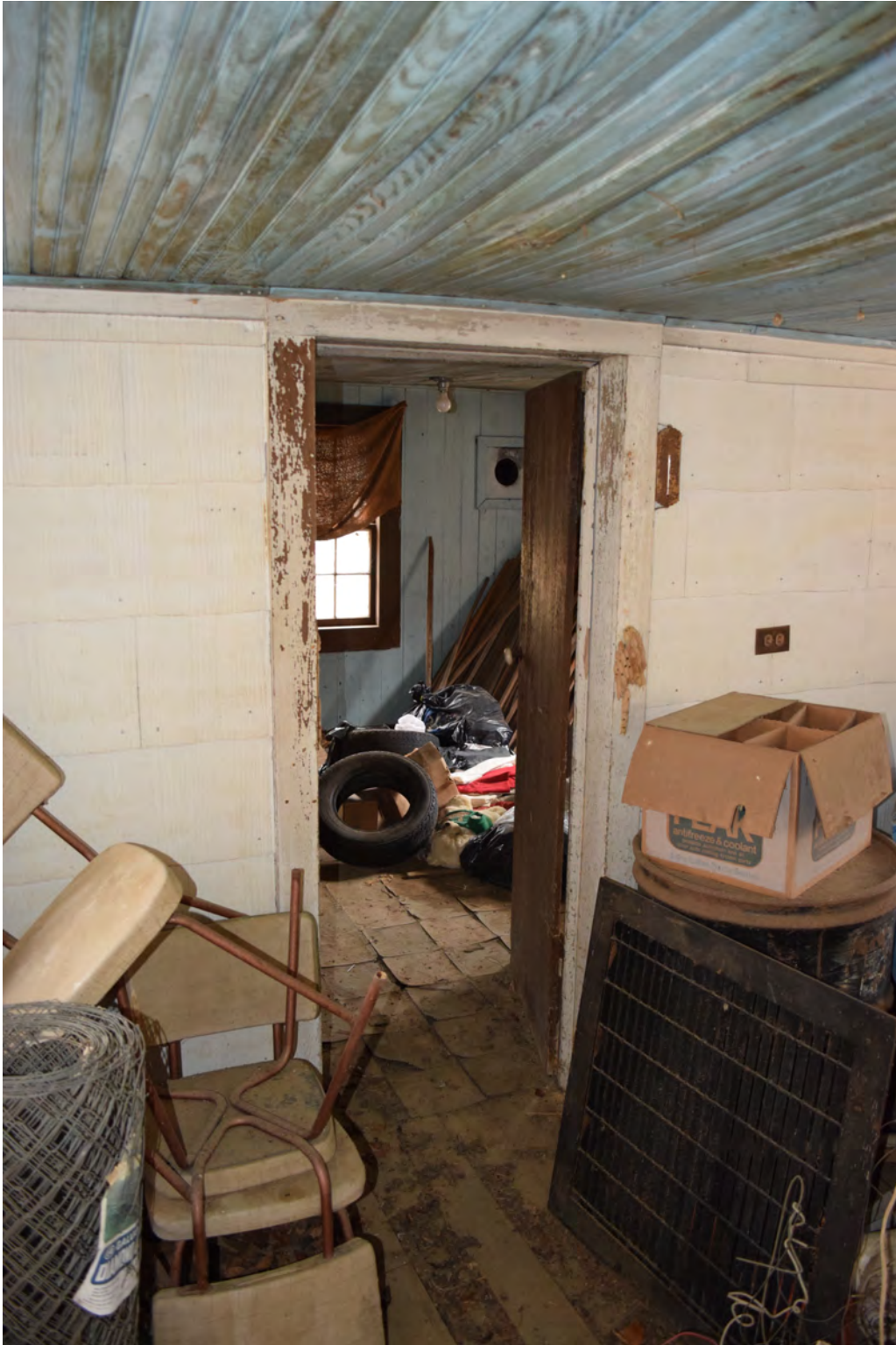
Figure 17: View into kitchen in addition, facing south-southwest
