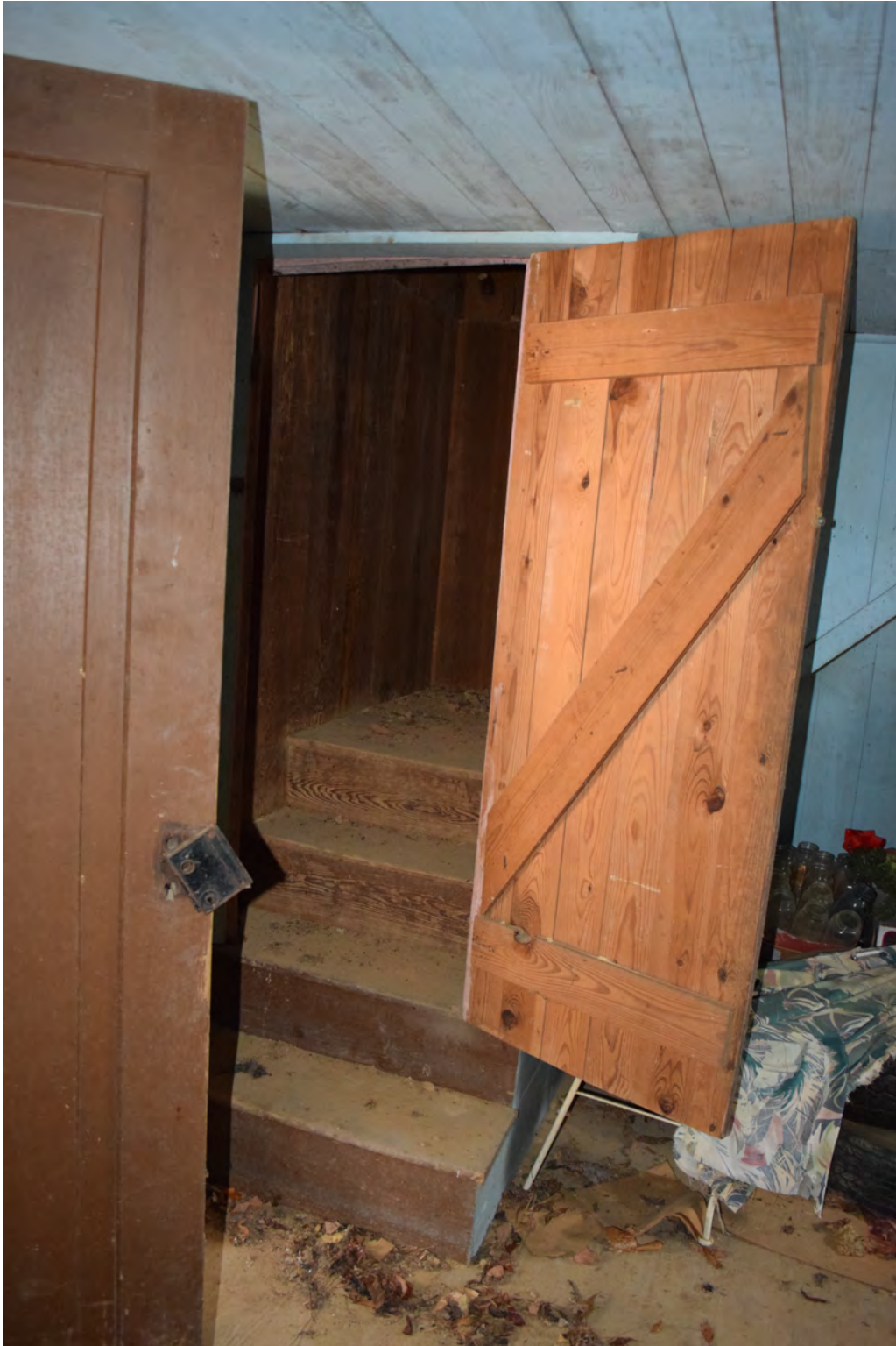
Figure 15: Boxed stair in southwest corner of original house, facing southwest
