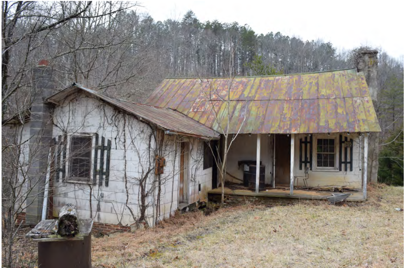
Figure 9: Tom Shelton House facade, facing northwest
