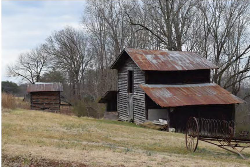
Figure 26: Outbuildings at the Moore Farm located at 2767 Moir Farm Road, facing east
