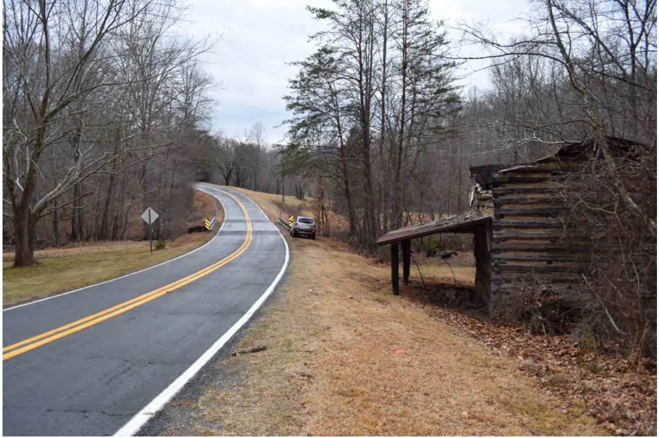
Figure 7: Tobacco barn north of bridge, facing south
