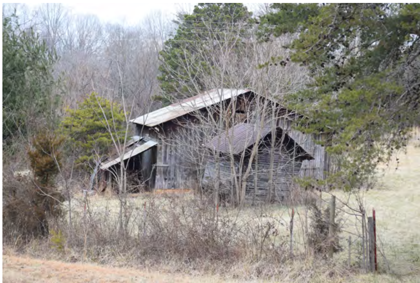
Figure 28: Outbuildings behind the John Elwood Priddy House
